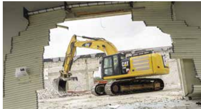
Demolition Day. Photo Credit: Tracey Benson Photography
